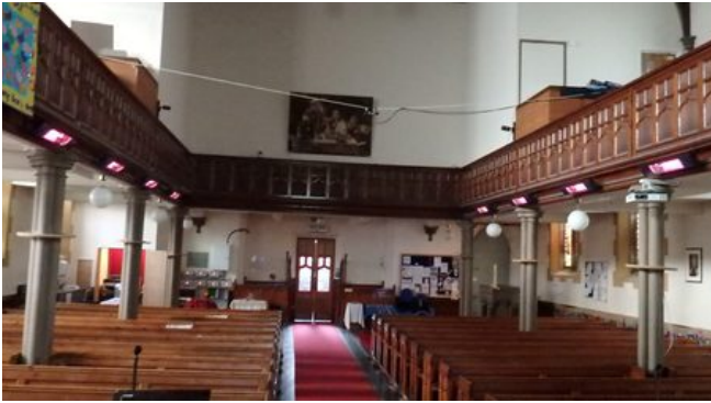
The galleried nave looking west. Timber galleries on three sides, stone columns and a large heated volume with no realistic route to insulation. These were the conditions that ruled out a heat pump.
