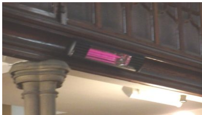
The same position in service. The emitter glow is visible but not glaring, and reads brighter here than to the eye, because the camera sensor is more infrared-sensitive than human vision.
